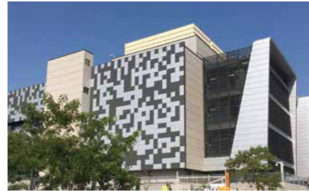
Global Switch Data Center / Hong Kong - Installed in 2018
