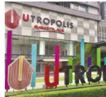
Paramount Utropolis / Malaysia - Installed in 2017
